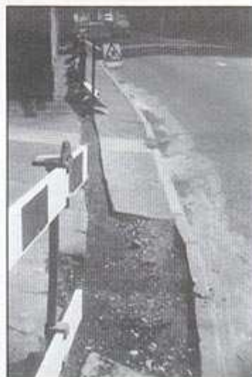
Only a narrow trench but...
