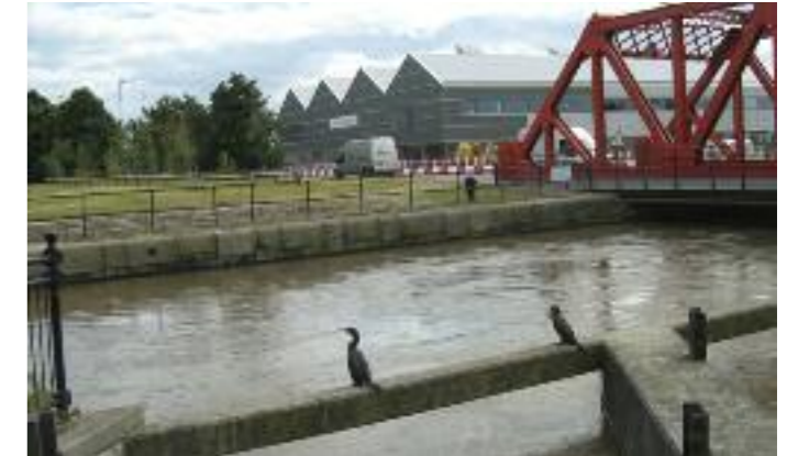
New Wirral Metropolitan College building, 12 Quays: photo - Rod Tann
